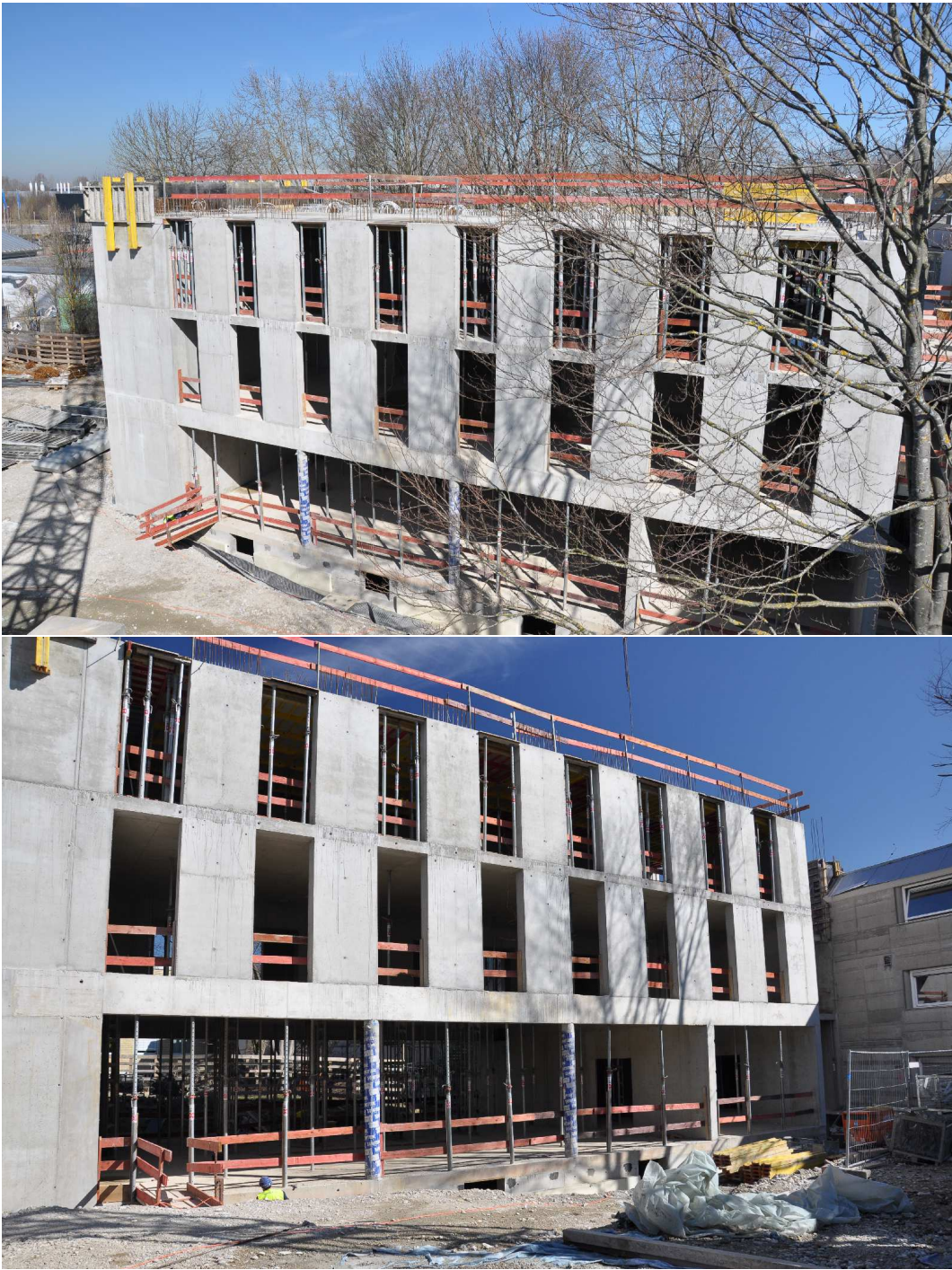
Figure 1.2: Construction of the MPA extension building/March 2012
