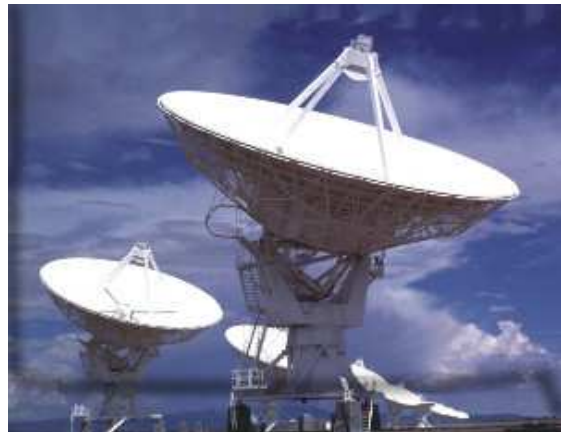
Figure 2.13: The Very Large Array (VLA) is a collection of 27 radio antennas located on the plains of San Augustin near Socorro, New Mexico, each with a dish 25 meters in diameter and weighing more than 200 tons. The data from all antennas can be combined electronically so that the array effectively functions as one giant antenna. Credit: NRAO/AUI
